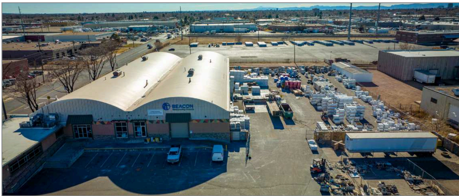
4343 Holly St. is 36,781 square feet on 3.65 acres and is leased to Beacon Roofing.
